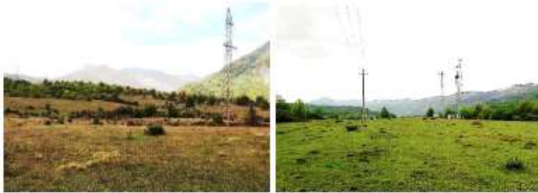
Picture 6. General Views of Camp #2 and Concrete Plant #2 Site
