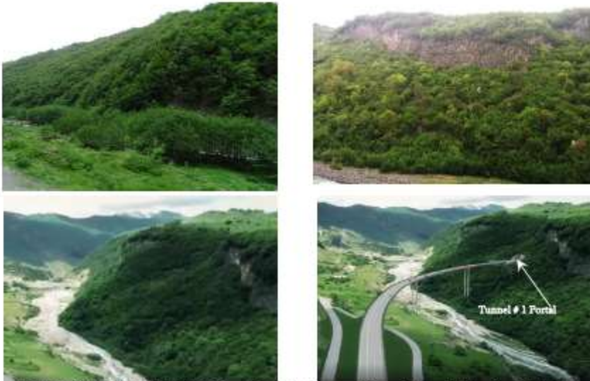
Picture 4. General Views of the site, view of the site after completion of the project (on the right, below)
