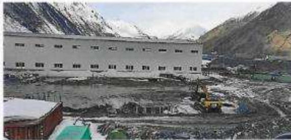
No drainages system on segment plant and batching plant area, the territory is flooded
