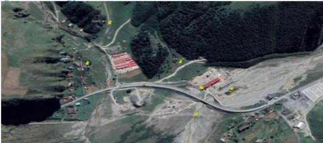
Image 2.1.2 Monitoring points on Kobi-Kvesheti Construction site
