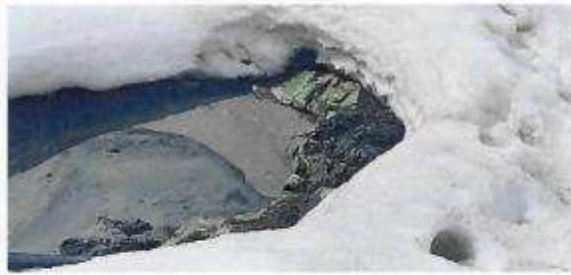
Groundwater collection pipe (near tunnel portal approximate coordinates X459372 Y4711527)
